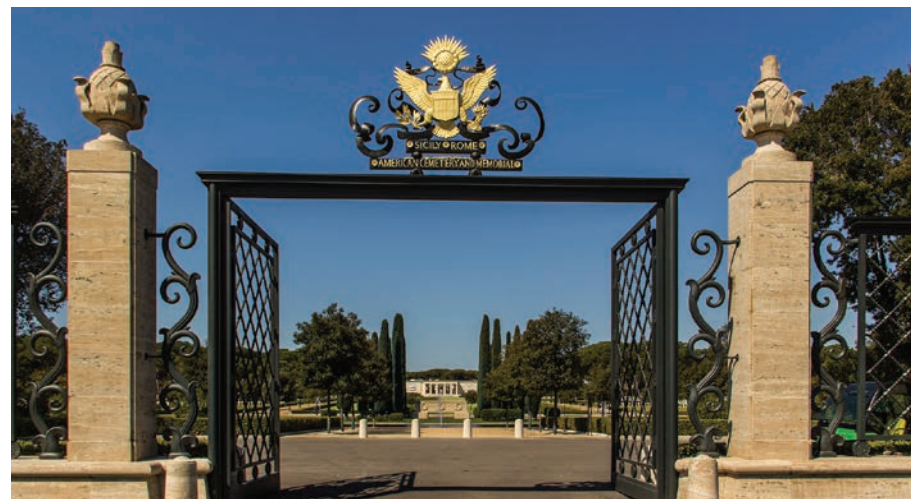
The U.S. seal surmounts the cemetery’s entry gates. Immediately inside to the right are the visitor building and the visitor center. (ABMC photo/Rich Arseneault)
