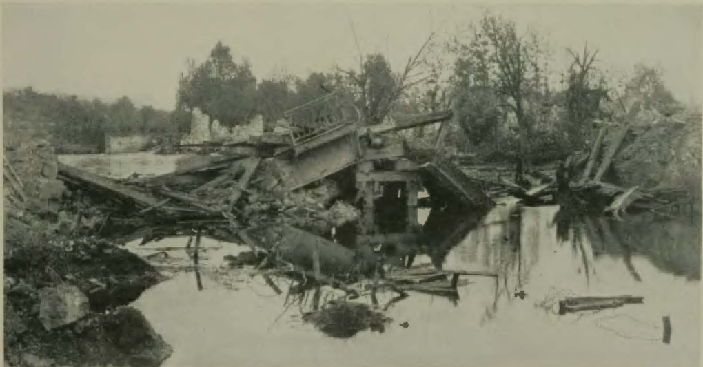
Main Bridge Between Fismes and Fismette Destroyed by the Retreating Germans
